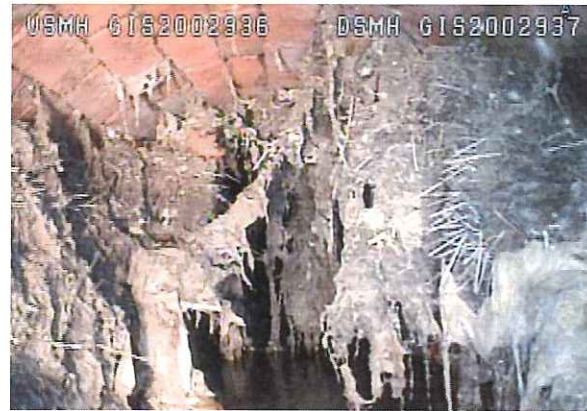
Old North Branch Interceptor Hartford
